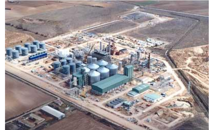
Abengoa Bioethanol facility
